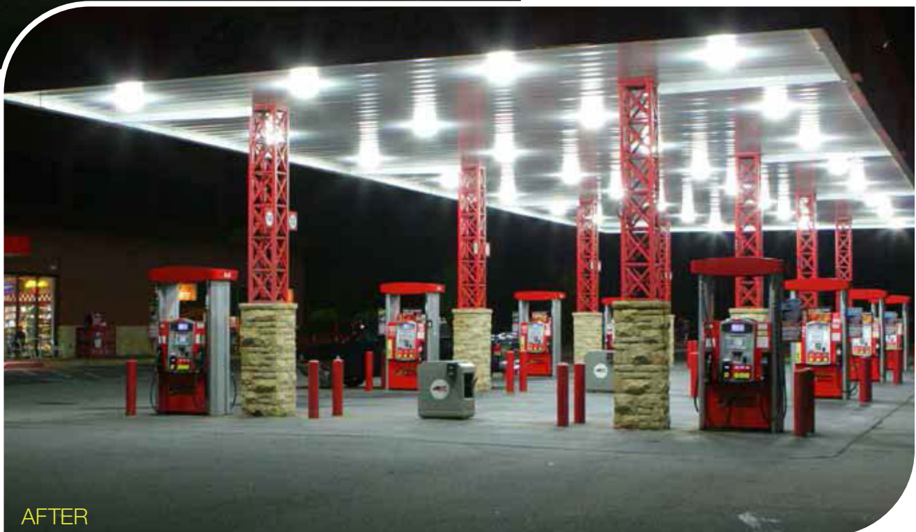
Example fixture after Retrofit Kit installation.
